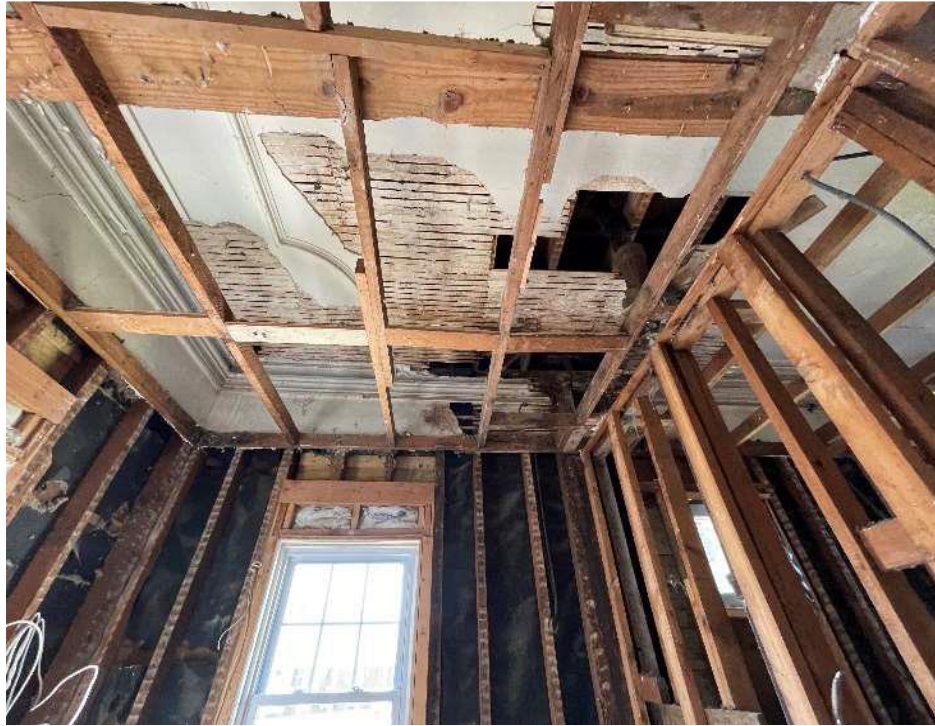
Photo 05: View of the second-floor ceiling joists and roof framing above.
